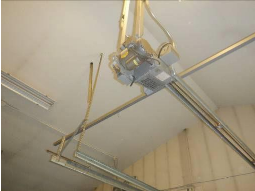
Ceiling suspended heater
