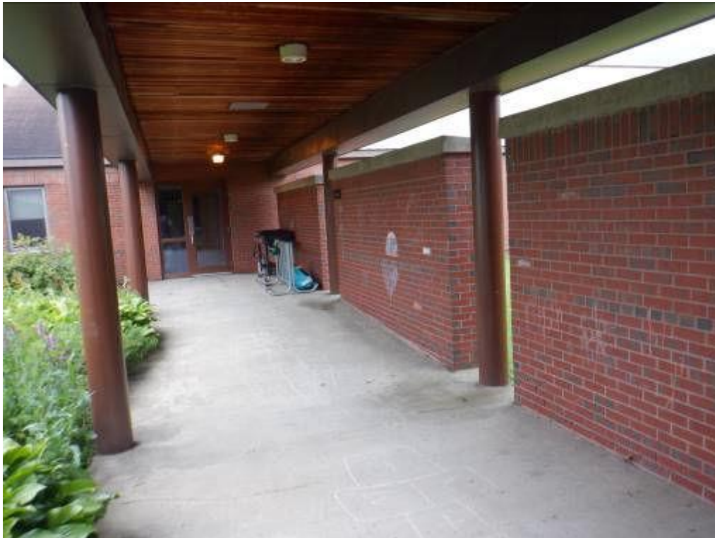
Interior of Connector, facing West to faculty apartment building. Finished and lighted ceiling, concrete slab.
