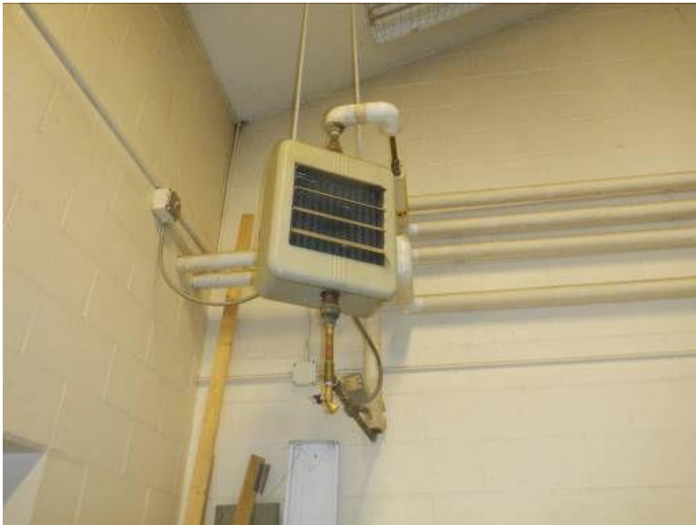
Ceiling suspended heater
