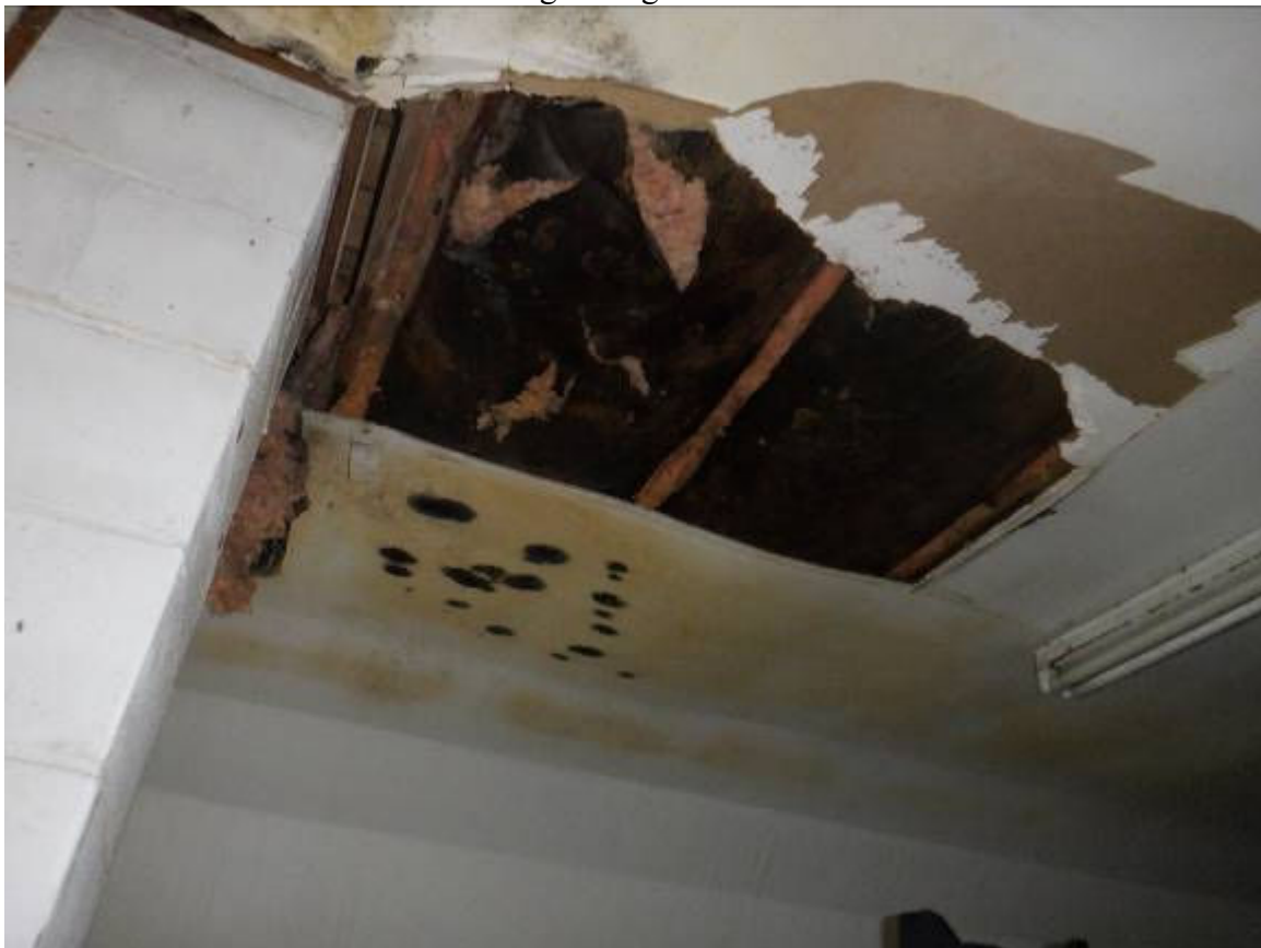
Ceiling damage and mold
