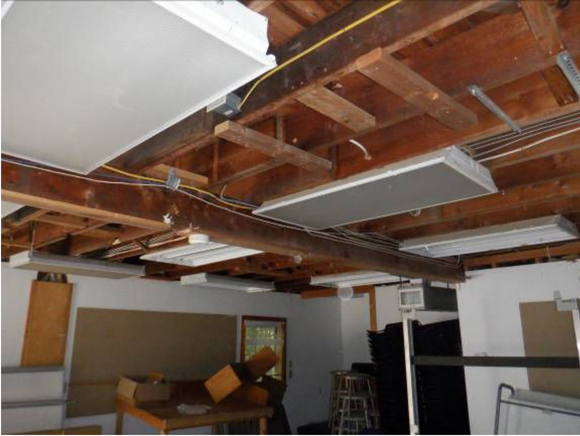
North section ceiling
