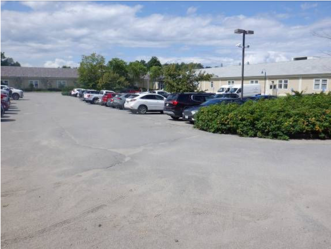
South and west walls
