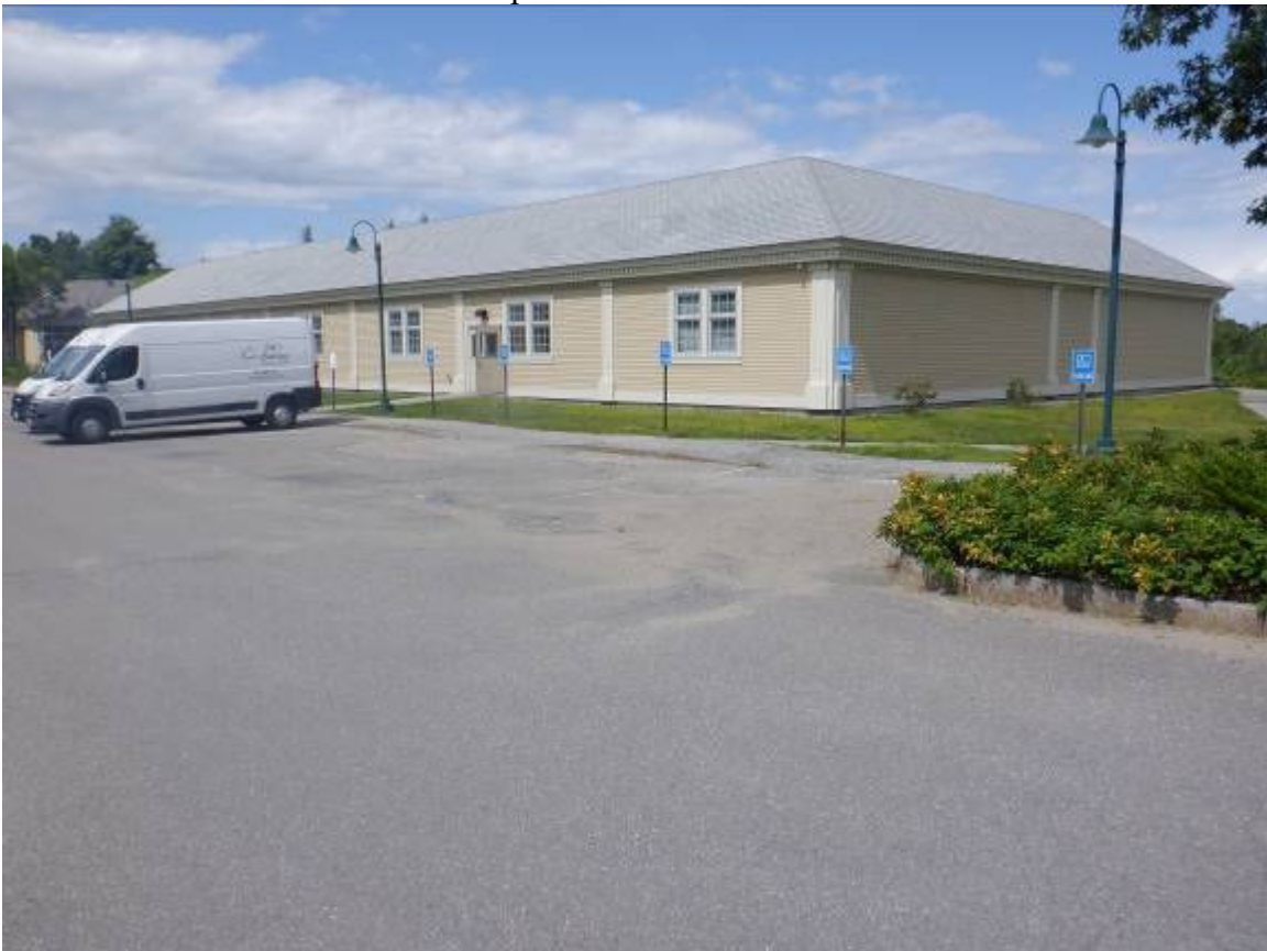
Close up of south and west walls
