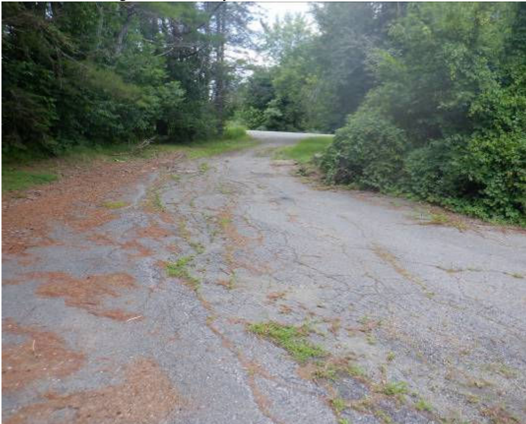
Facing north, driveway to the Barn from Belmont Avenue
