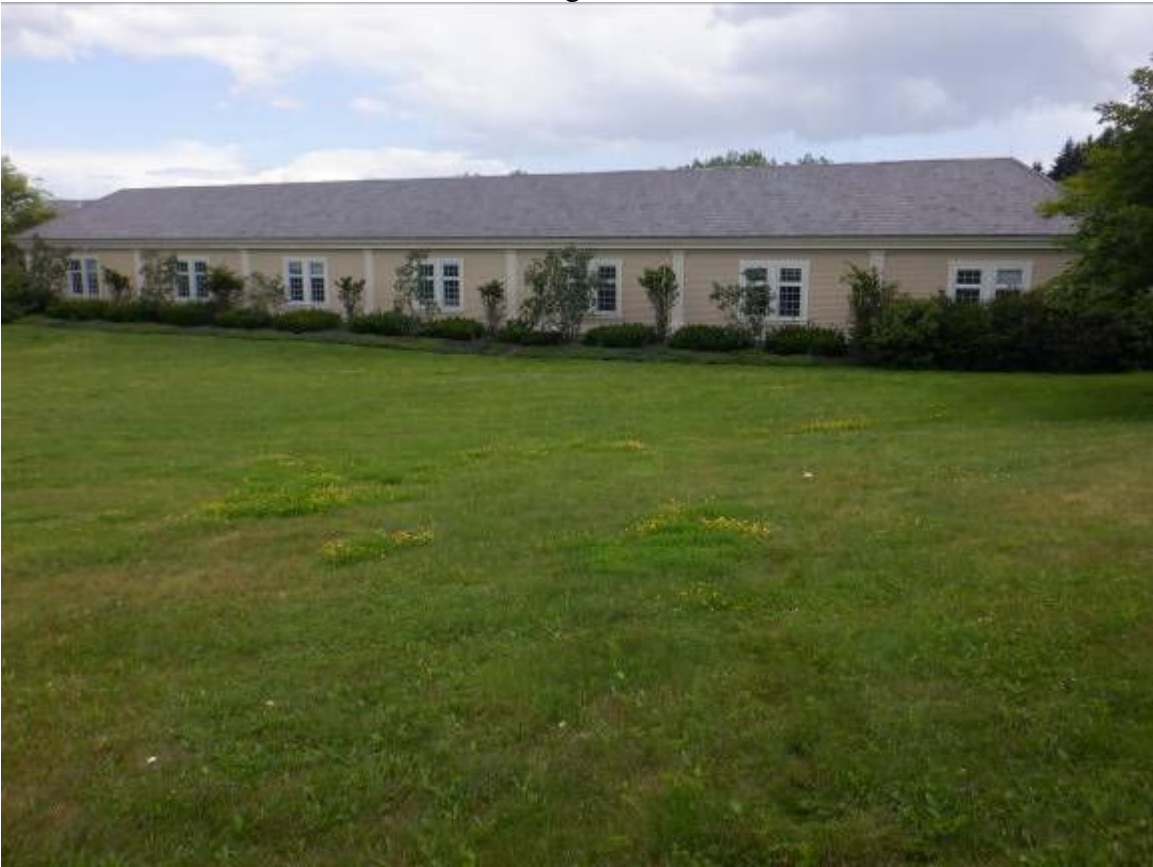
North wall, facing Belmont Avenue
