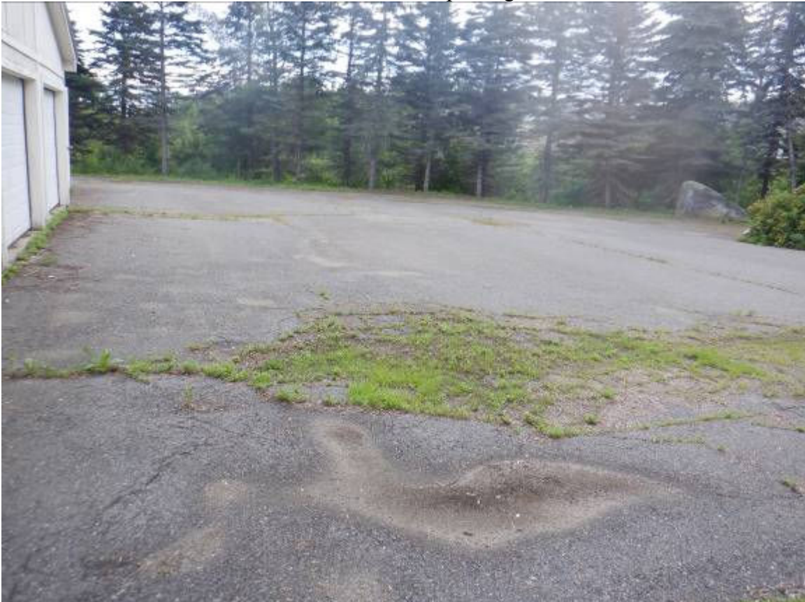
West section of the parking lot
