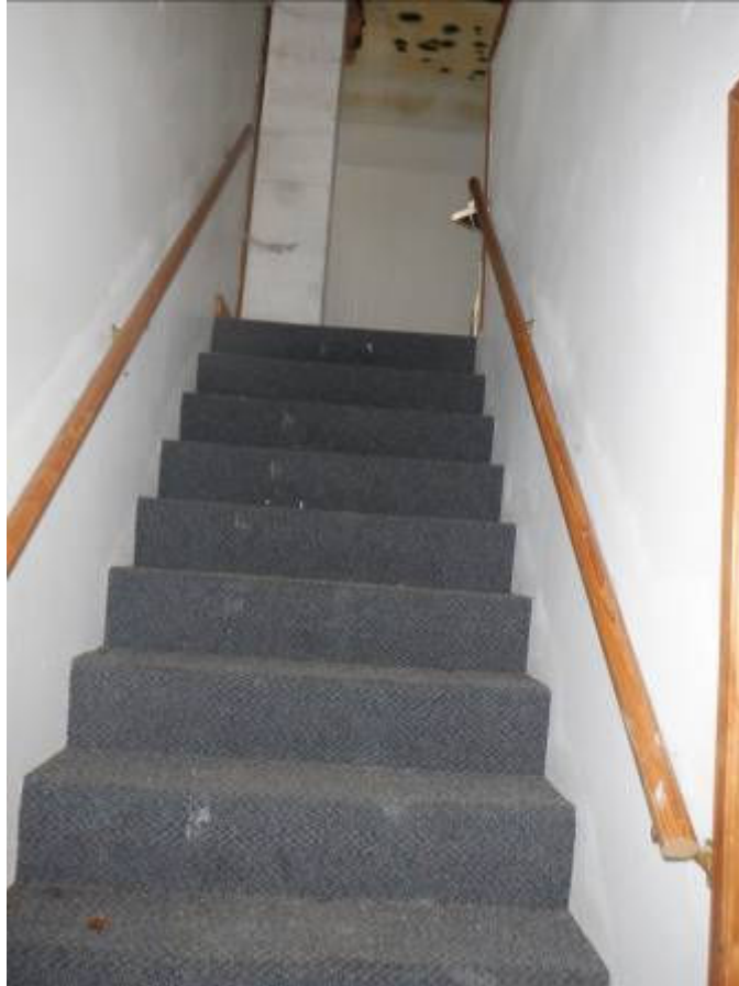
Ceiling damage and mold
