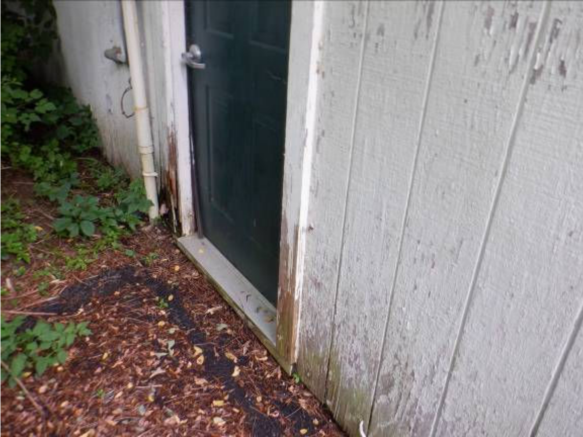
North wall passage door.
