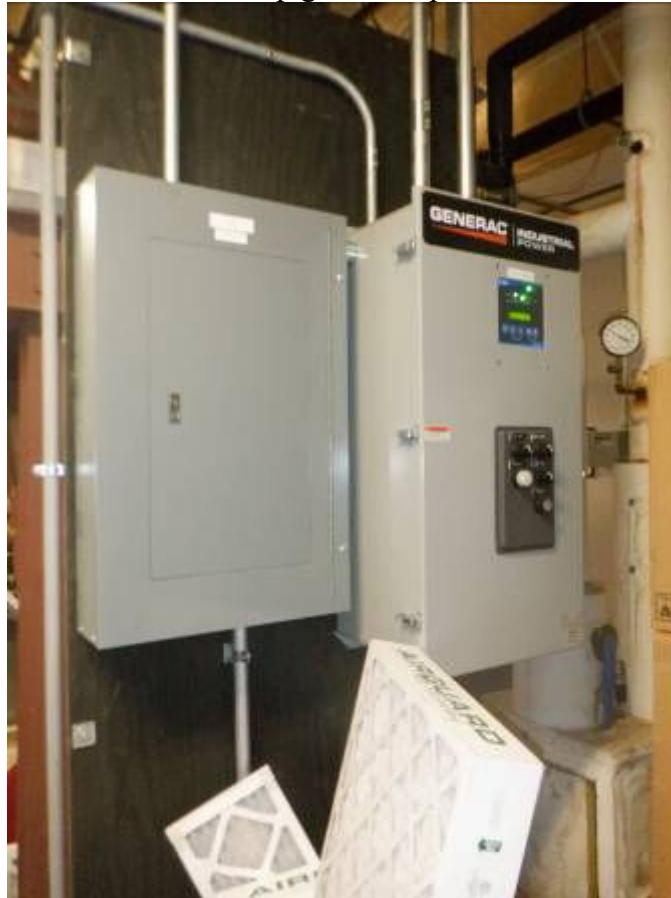
Back up generator panel
