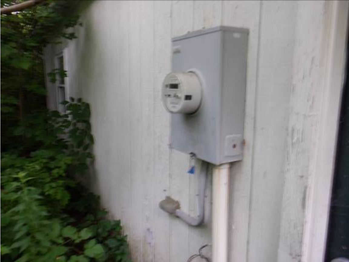
North wall of the barn
