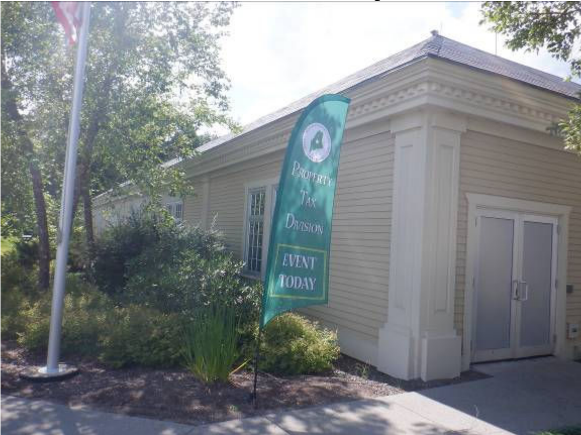
South wall of the west wing
