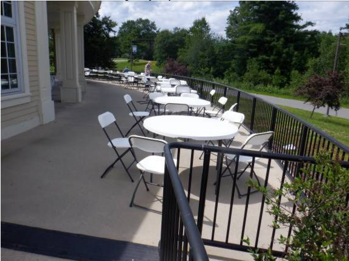
View of good quality outside concrete deck
