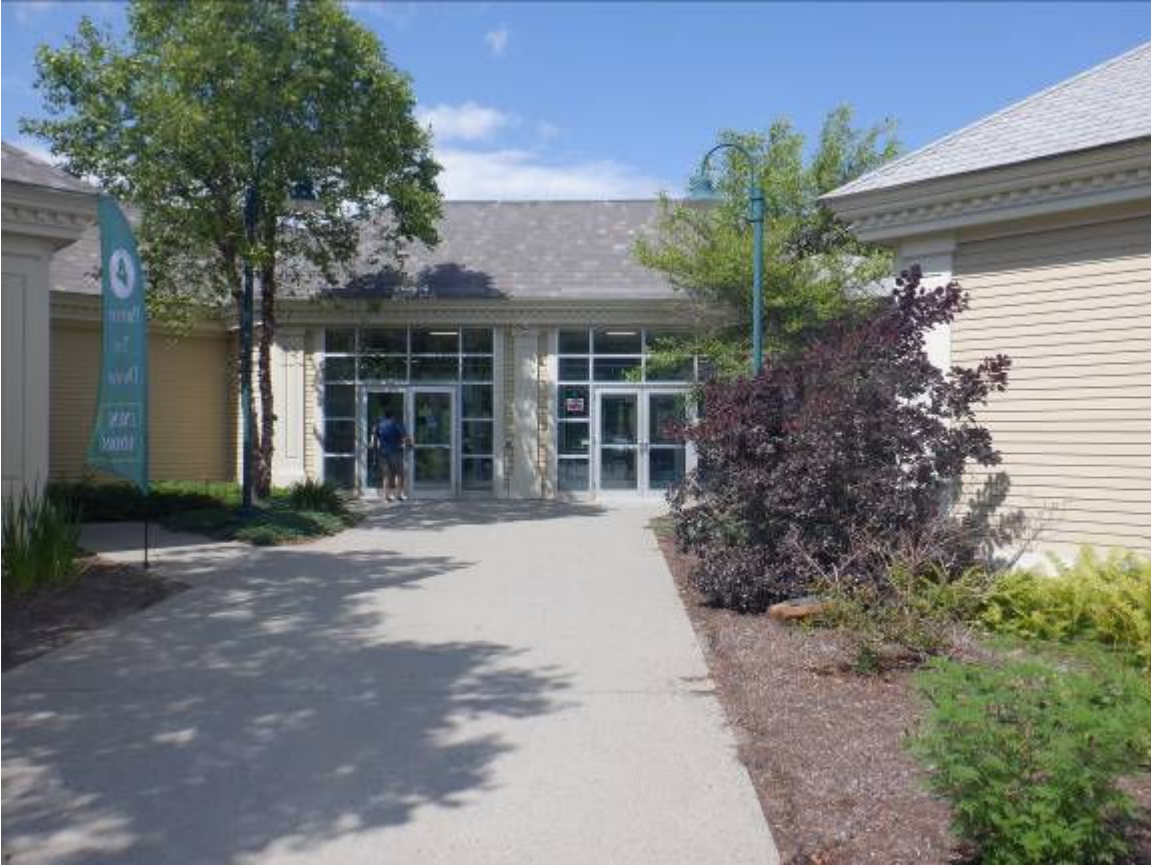
Main entrance on the south wall
