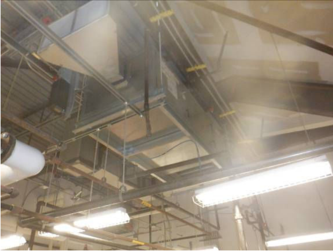
Another view of the steel framing and decking
