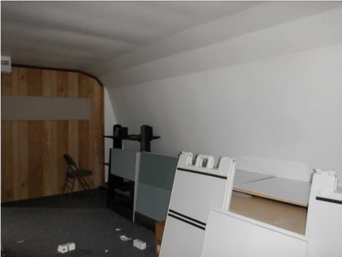
Second floor, north wall
