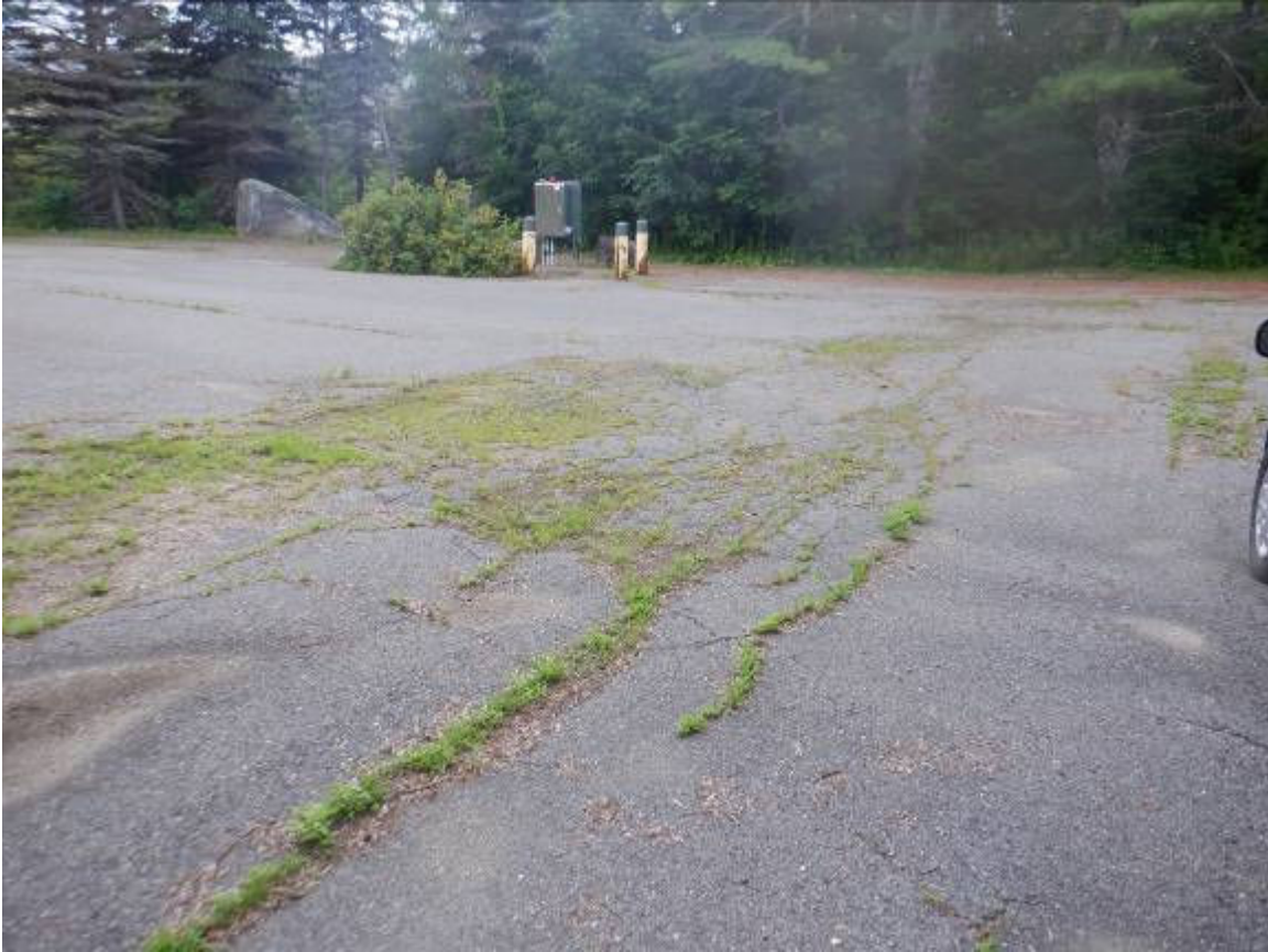
Paved area on the west section of the parking lot
