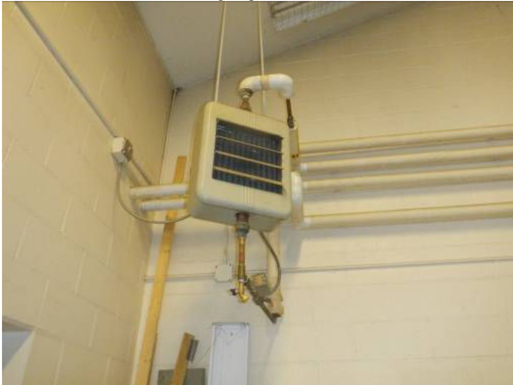
Ceiling suspended heater
