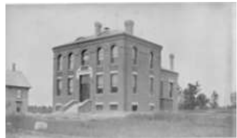
Figure 6: Holmes Hall original construction
