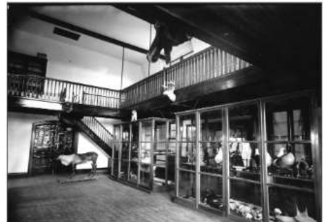
Figure 5: Coburn Hall Interior
