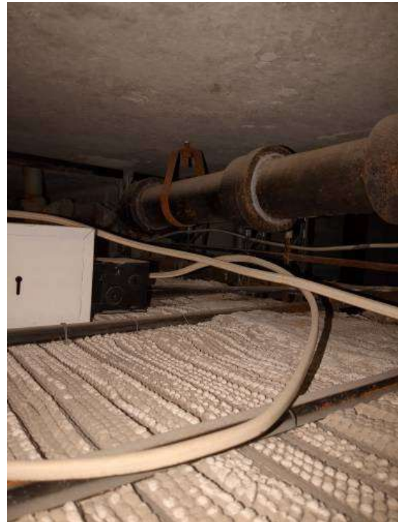
View of plumbing inside Shower Soffits – No pipe insulation observed
