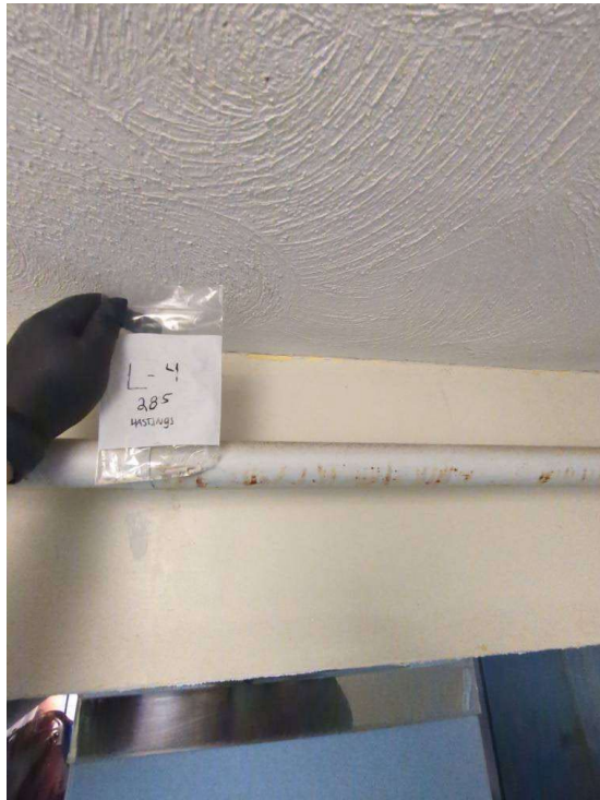
Hastings Wing Bathroom 285; Off-White/Yellow Soffit Paint
