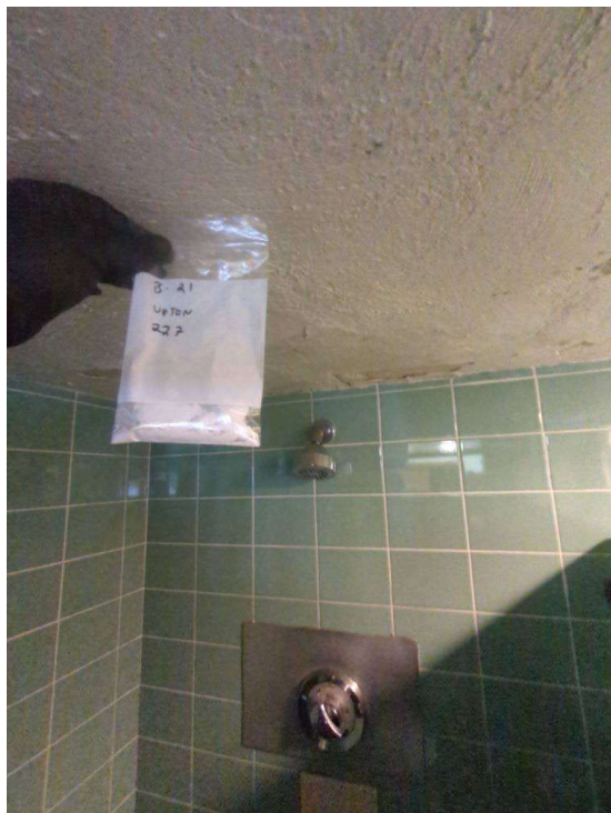
Upton Hall Core Bathroom 227; Shower Stall Ceiling Texture
