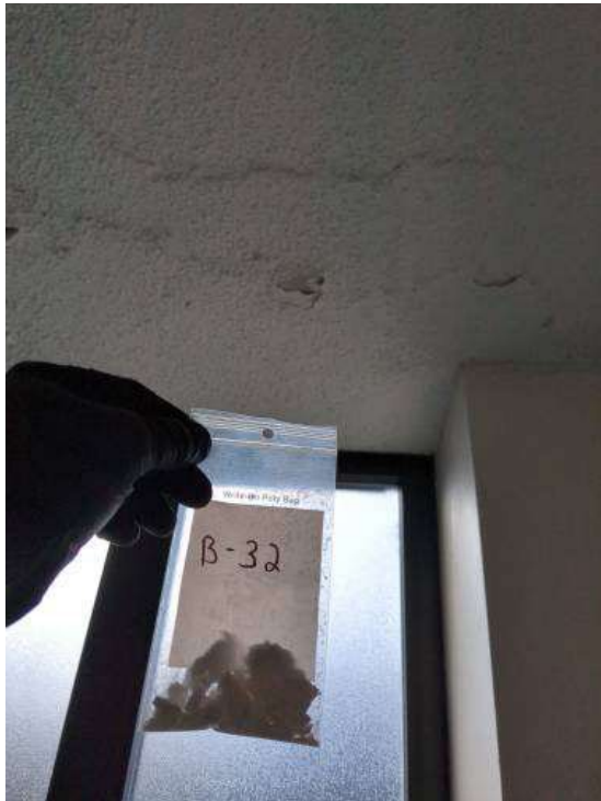
Hastings Women's Core Bathroom 476; Ceiling Texture
