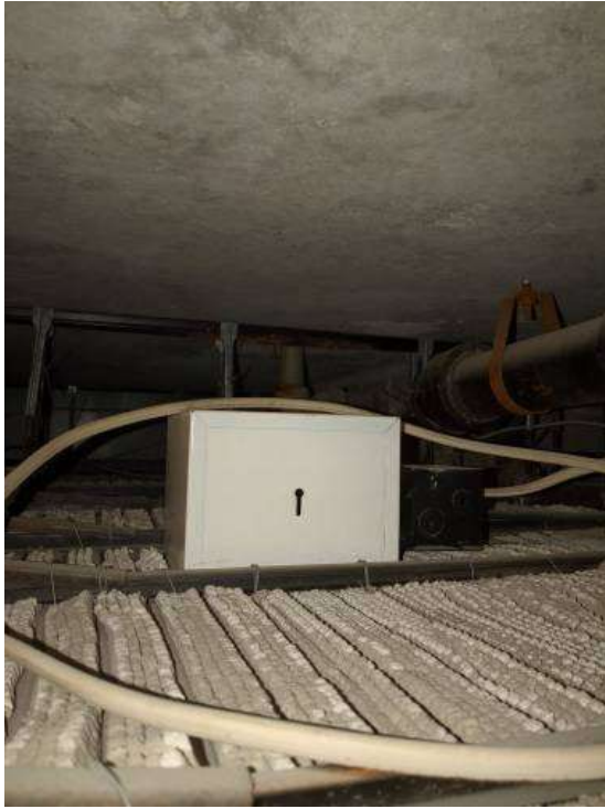
View of plumbing inside Shower Soffits – No pipe insulation observed
