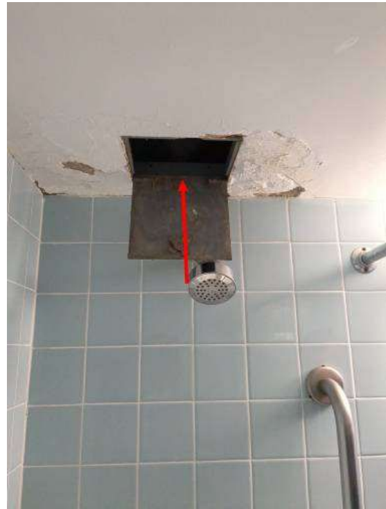
Hastings Core Bathroom 277; Shower Stall Ceiling Plaster (Base Coat)
