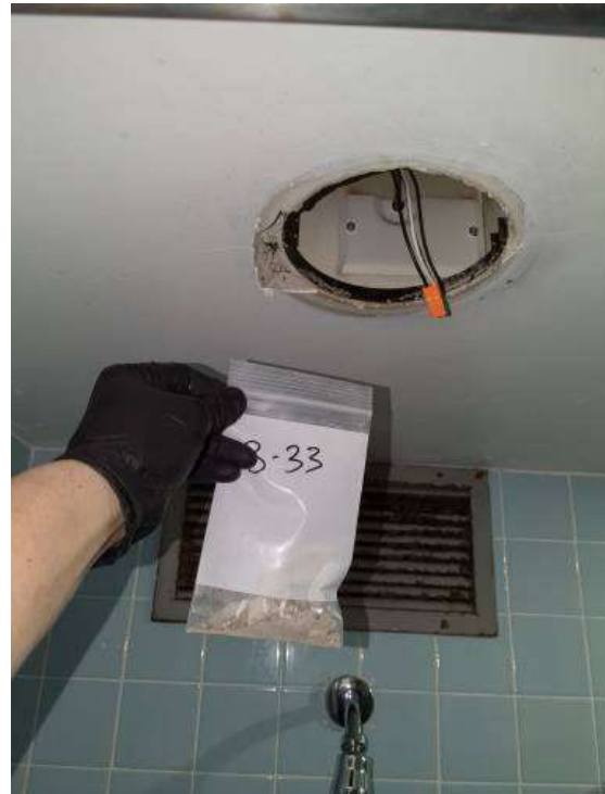
Hastings All Gender Wing Bathroom 480; Shower Ceiling Plaster
