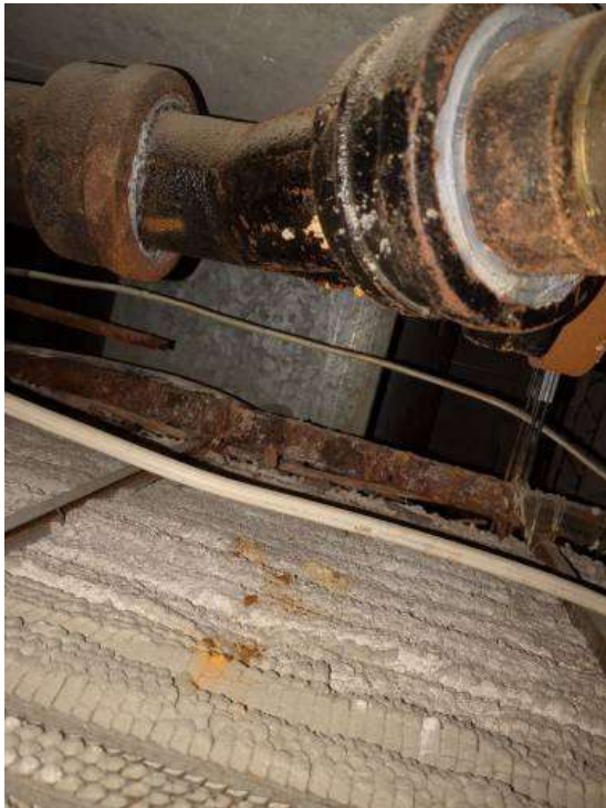
View of plumbing inside Shower Soffits – No pipe insulation observed
