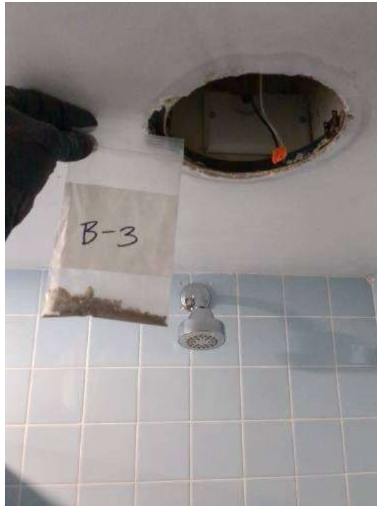
Hastings Core Bathroom 277; Shower Stall Ceiling Plaster (Base Coat)
