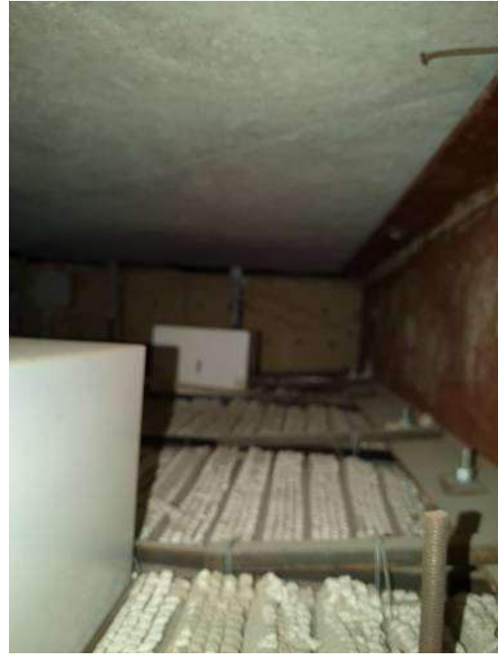
View of plumbing inside Shower Soffits – No pipe insulation observed
