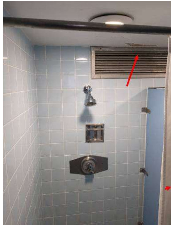
Hastings Core Bathroom 277; Shower Stall Ceiling Plaster (Skim Coat)
