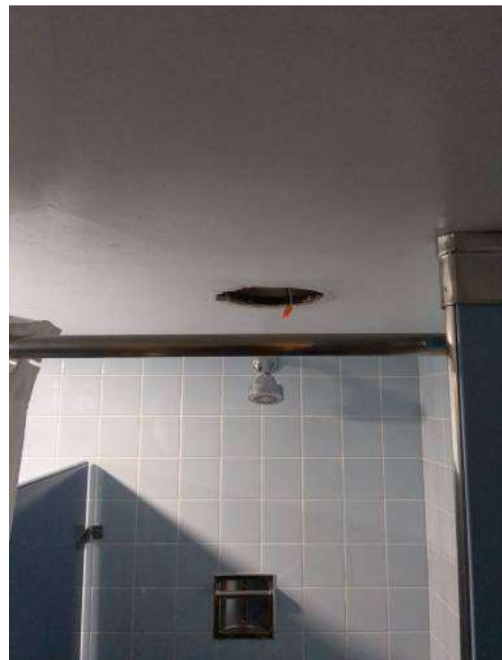
Hastings Core Bathroom 277; Shower Stall Ceiling Plaster (Skim Coat)
