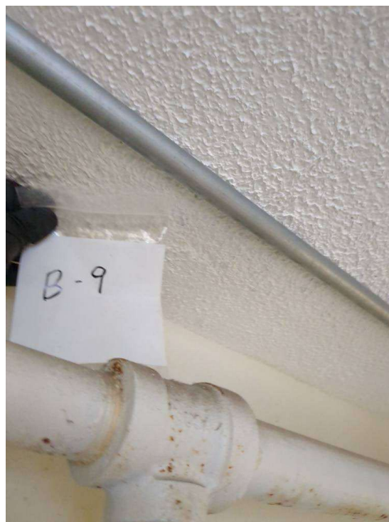
Hastings Core Bathroom 277; Ceiling Texture abutting Soffit
