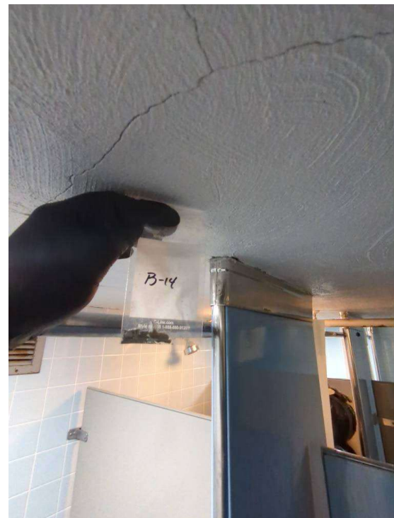
Hastings Wing Bathroom 285; Shower Stall Textured Plaster
