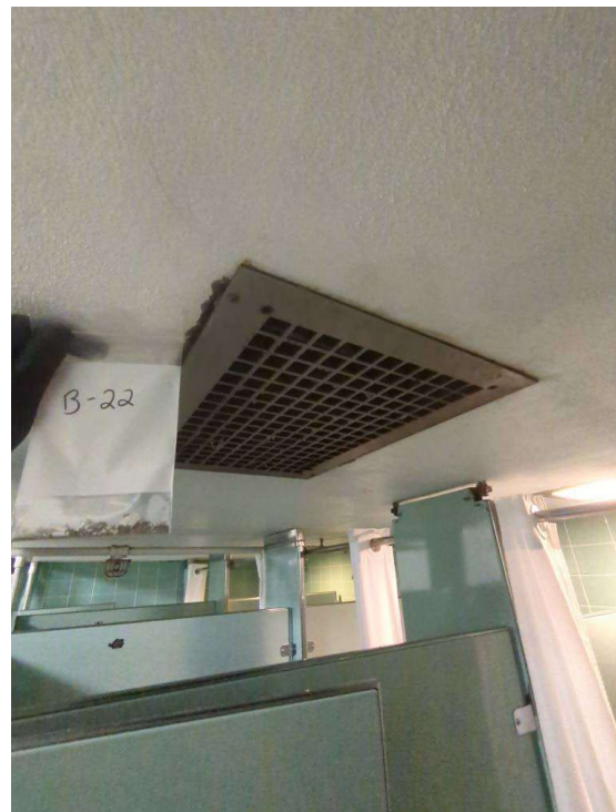
Upton Hall Core Bathroom 231; Shower Stall Ceiling Texture
