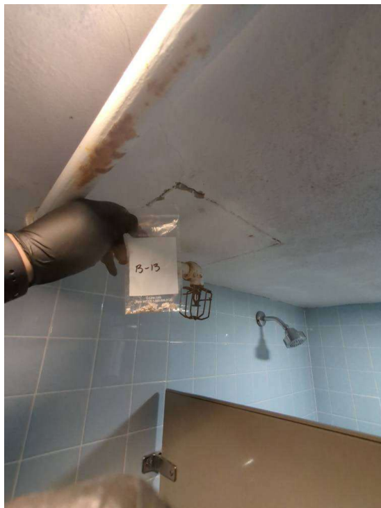
Hastings Wing Bathroom 285; Shower Stall Textured Plaster
