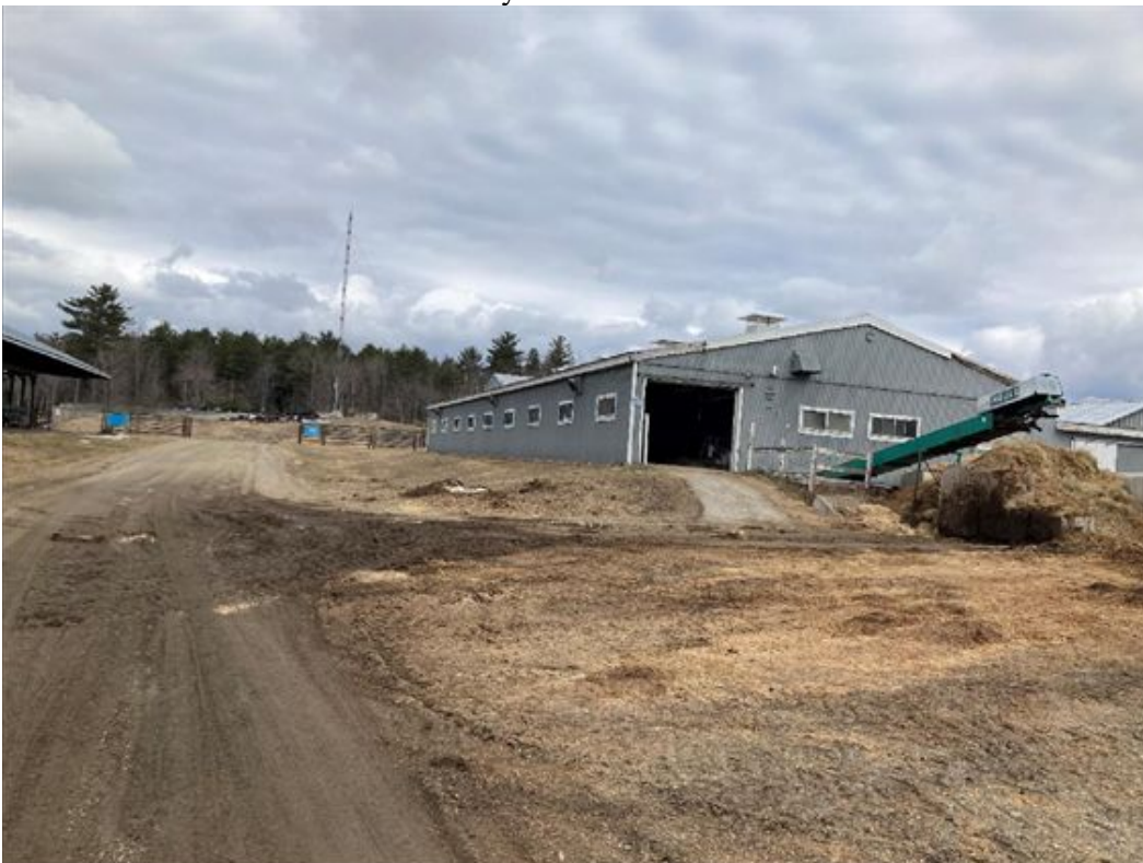
Current Dairy Barn to be demolished
