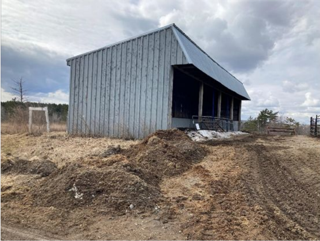
Sheep Shed to be demolished.
