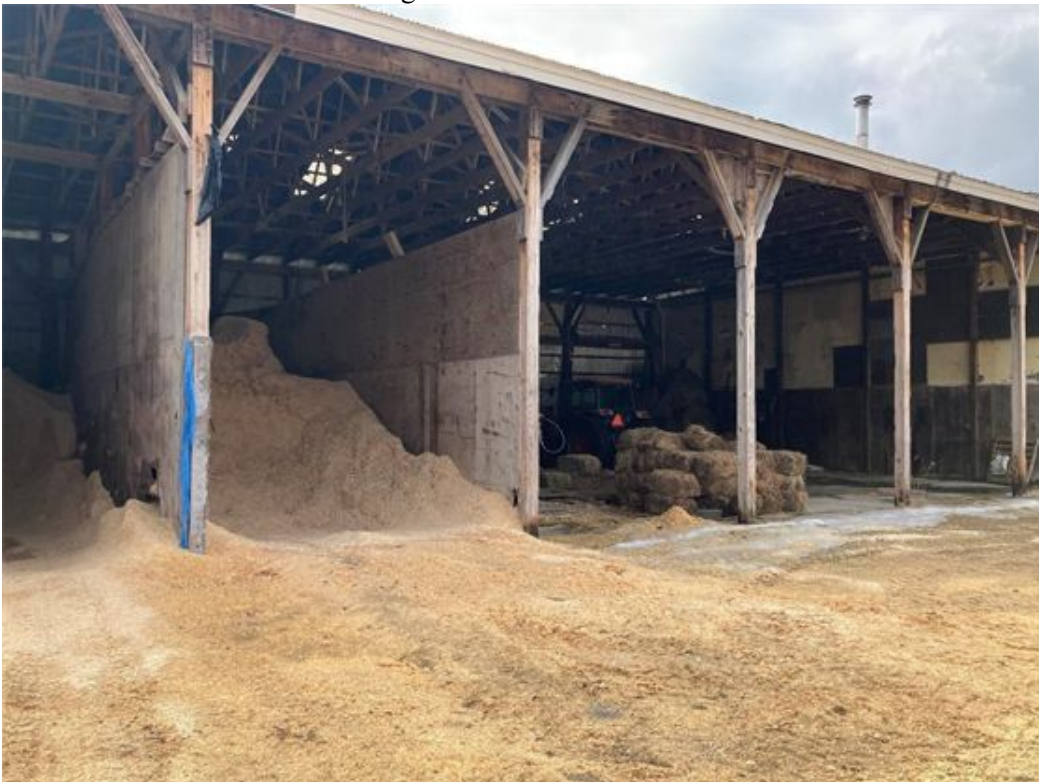
Storage Barn to be demolished.
