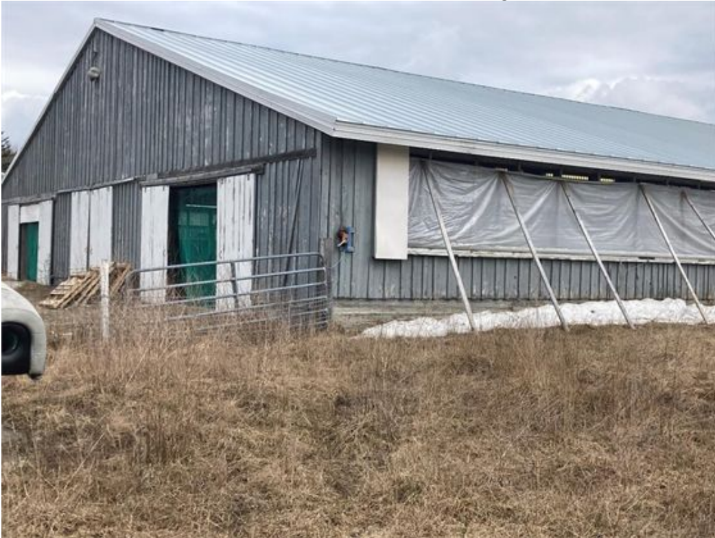
Current Horse Barn to renovate into Storage Barn
