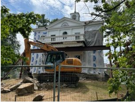
Overall view showing portico temporarily supported Foundation being excavated
