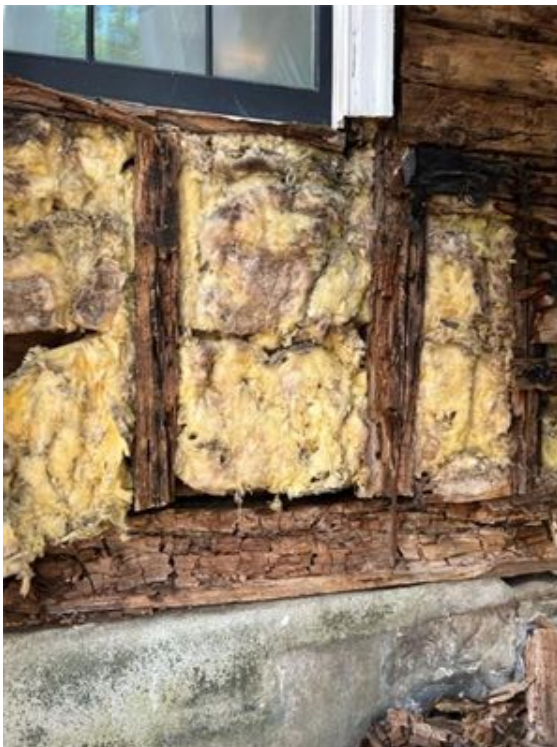
Sill and wall framing @ south window 1 st floor (Outside corner)
