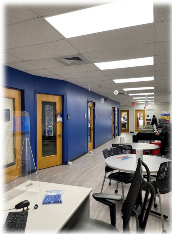
Katz Library – Student Support and TRiO Scholars renovation
