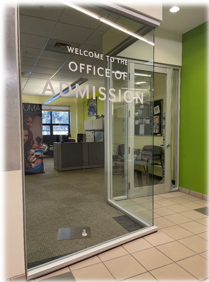
Admissions Office Renovation
