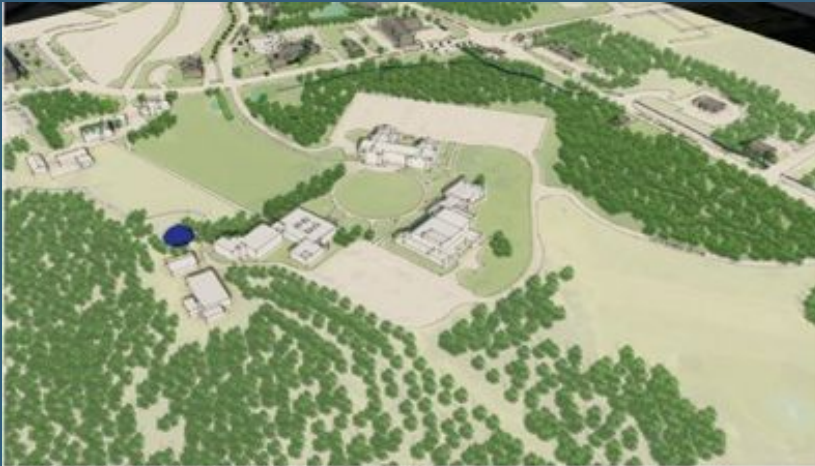
Figure 0.18 Augusta Campus Existing Conditions, Looking Northwest
